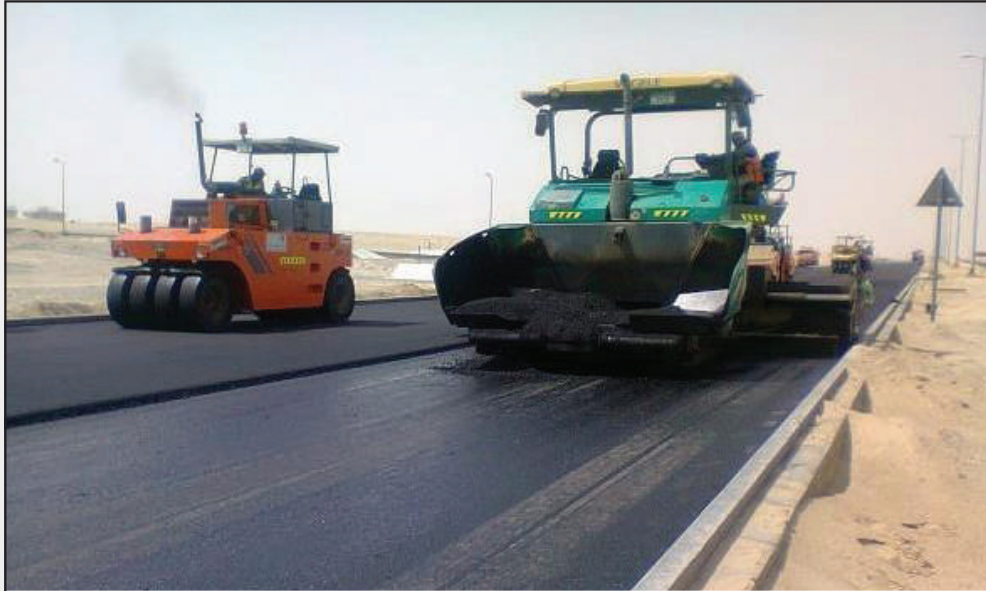
Strengthening and widening of existing 2- lane road to 4- lane dual carriageway from km 50 to 62.5 of NH-6 at Nagpur (MH)
