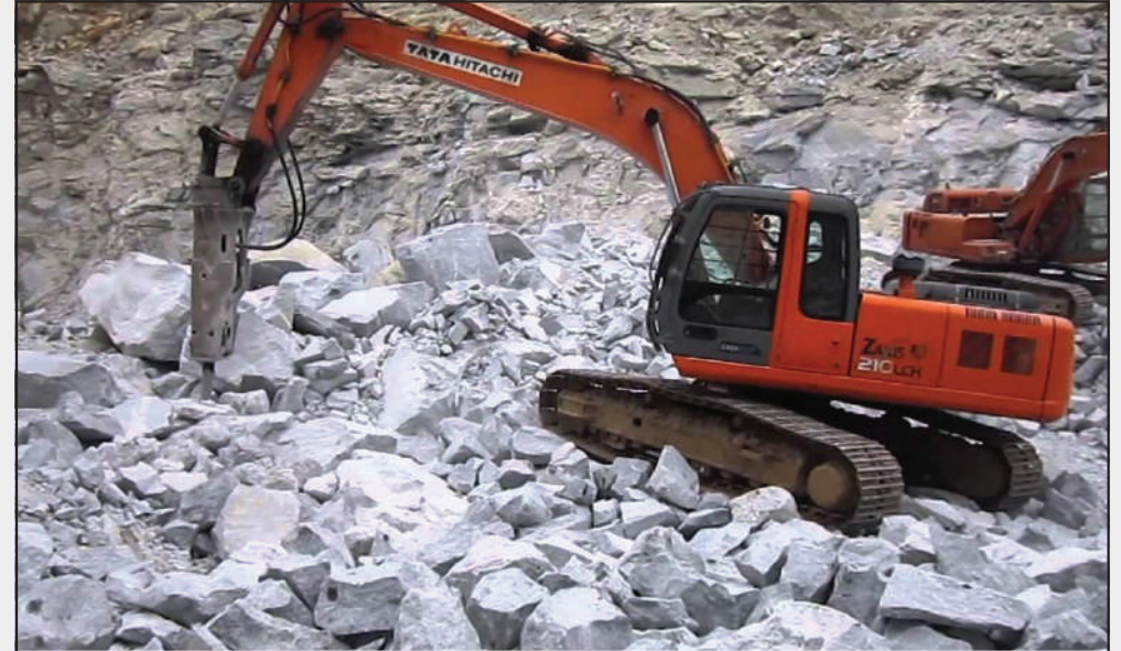
Earthwork in cutting to form formation and earthwork in filling to form embankment / sub-bank and construction of minor bridges, retaining wall, pacca approach road to allinment and other ancillary work between chainage km 49.2 to km 51.30
