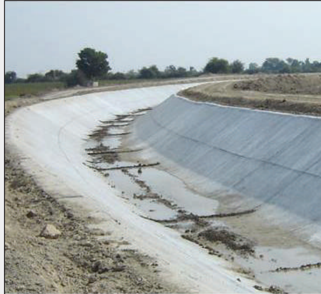
Construction of Earthwork, C.C. Lining, Structure and Road Approaches of distributaries of Jhinjhuwada Branch Canal
