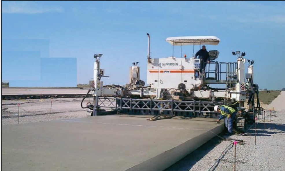
Construction of Manrol to Bagalwada Road Length 20.92 km under district Riasen
