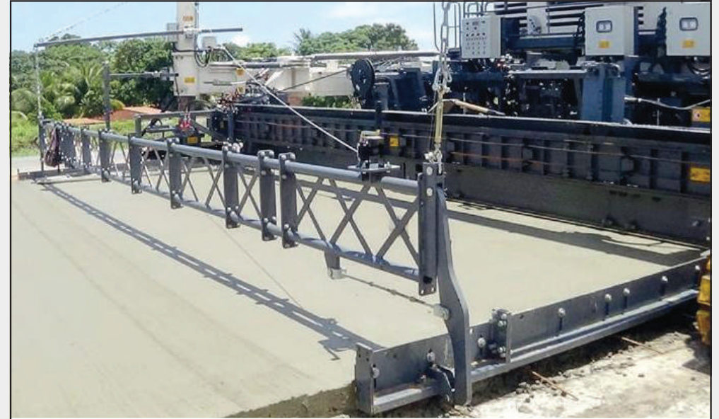
Construction Upgradation of Bangrasia-amjhara-bilkhiriya road (dist- bhopal) intermediate lane (5.5m) desing length-20.685 km
