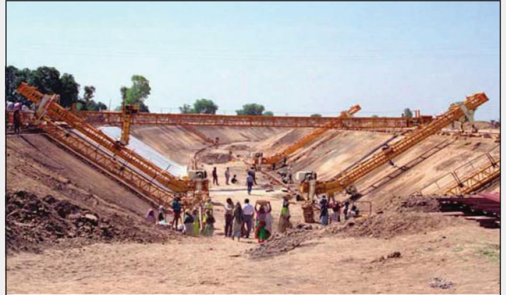
Construction of C.C. lining of Vallabhipur branch canal. Ch. 15.020 to 31.600 km ( package -2b )
