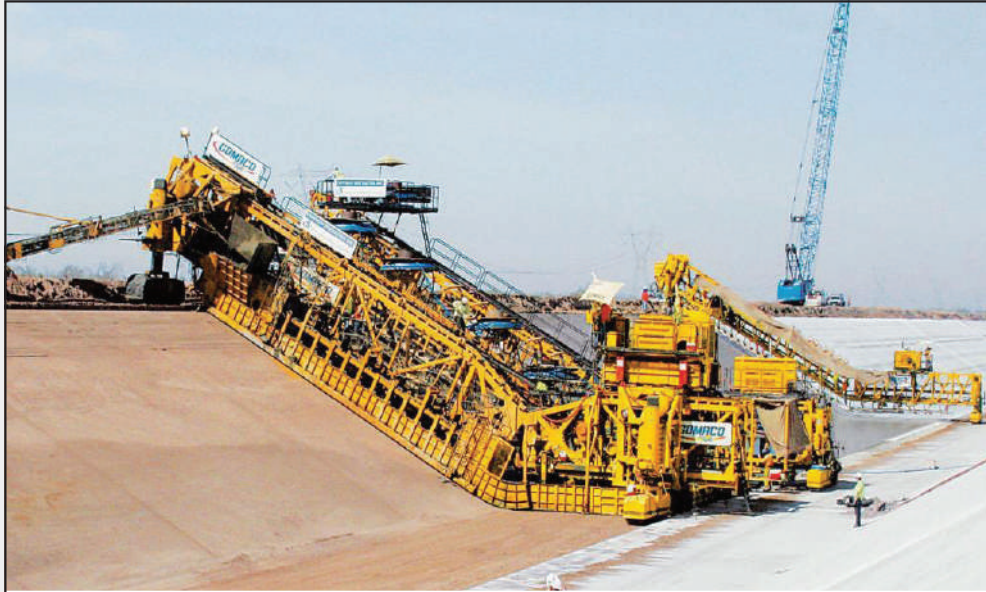
Improvement of existing irrigation Infrastructure work on Kosmaba Branch ch 0.00 km to 18.272 km Ex URBMC
