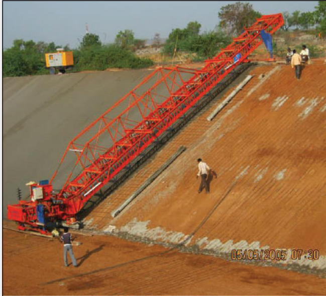
Constructing NMC Reach 362.476 km to 368.431 km (Slice-9b) Thara
