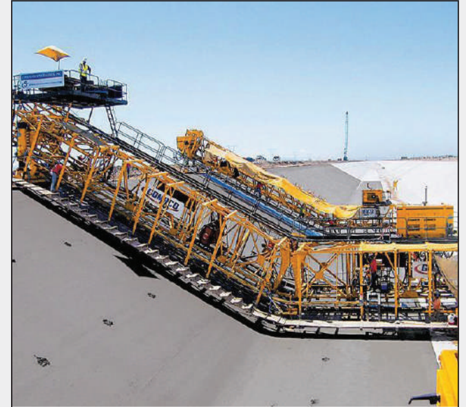
Improvement of existing irrigation Infrastructure work on Kosmaba Branch ch 18.272 km to 38.545 km Ex URBMC
