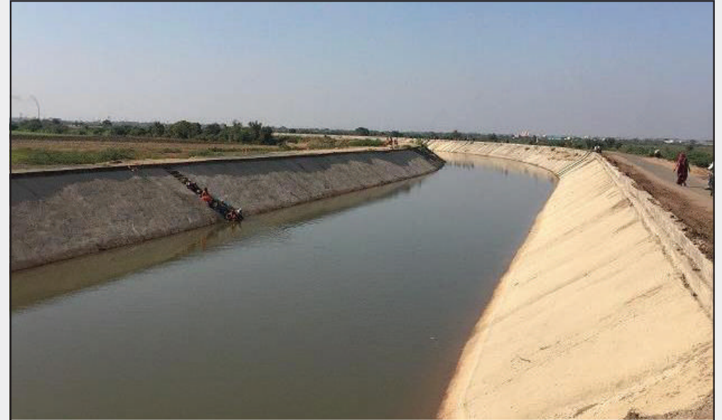
Constructing Canal earthwork and cement concrete lining on Saurashtra Branch Canal Ch. 82.140 to 85.725 km
